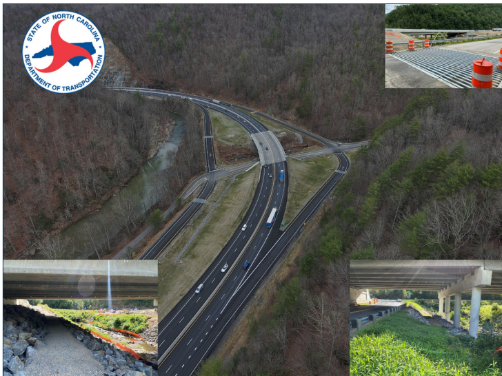
I-40 & COLD SPRINGS CREEK INTERCHANGE (EXIT 7, HARMON DEN) (NCDOT)
